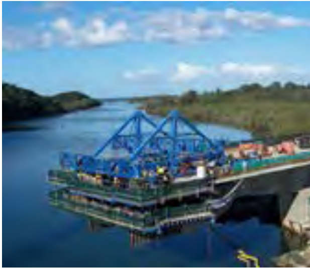
Figure 2.10 - Typical Balanced Cantilever Construction (Brunswick River, NSW)
